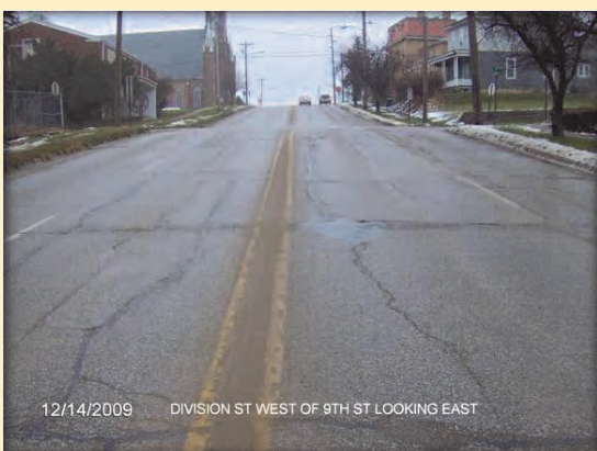
Burlington—Existing Division Street Surface
