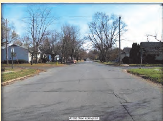
Fort Madison—Existing Ave E Surface
